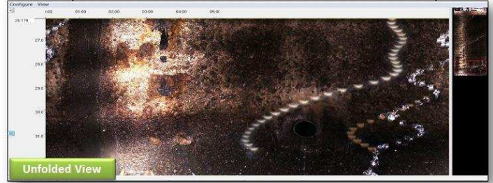
3D Optical Manhole Scan 2- FS020104 Front St at Poplar
