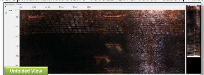
3D Optical Manhole Scan 3- FS031142 Front St at Peabody Place
