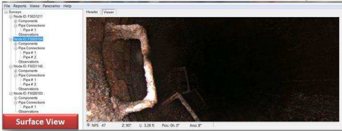
3D Optical Manhole Scan 2- FS020104 Front St at Poplar
