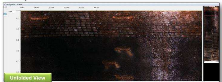
3D Optical Manhole Scan 1- FS031211 Front St at Butler Ave
