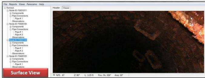
3D Optical Manhole Scan 3- FS031142 Front St at Peabody Place
